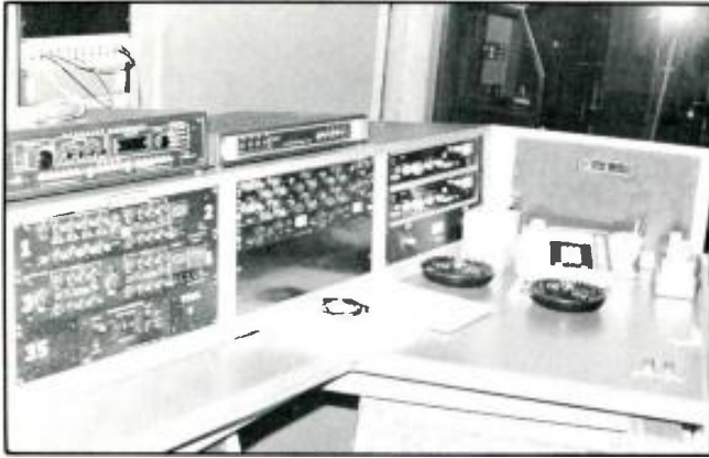
A closeup of the equipment rack.
